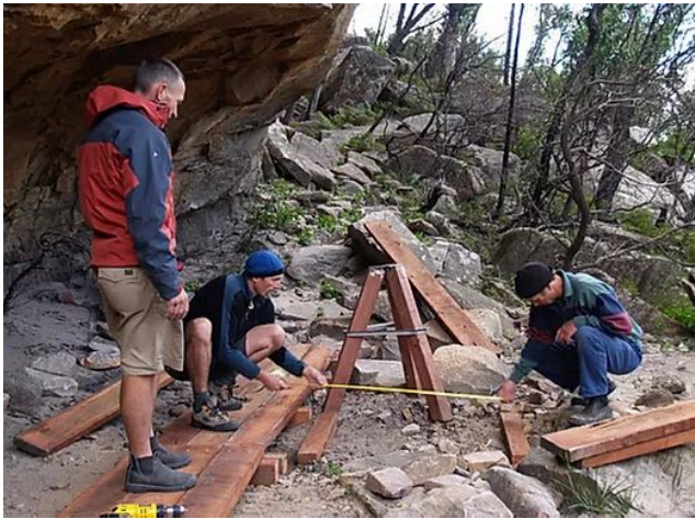
Pic 7 and 8. In 2008 after Aboriginal Surface Scatters were discovered under a climb named “Manic Depressive” at Bundaleer, CliffCare and Parks Victoria’s Cultural Heritage team worked together to create a boardwalk and wooden tripod to protect both this area and the climb above. Photo Credit Cliffcare Collection
