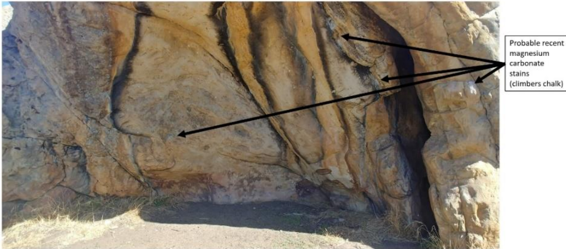
Figure 14A: Evidence of chalk stains from Rock Climbing on the boulder. R. Cayley, GSV, June 2020
